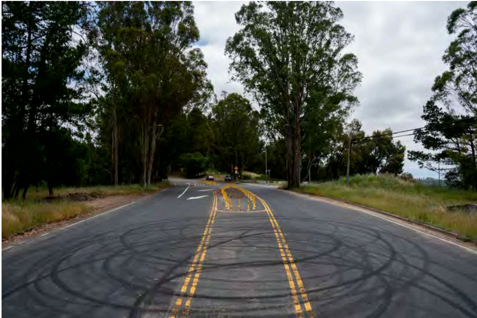
Despite the addition of bollards and hard centerlines in the roadway in 2021, the intersection of Keller Avenue and Skyline Boulevard remains a popular sideshow spot. Credit: Florence Middleton
