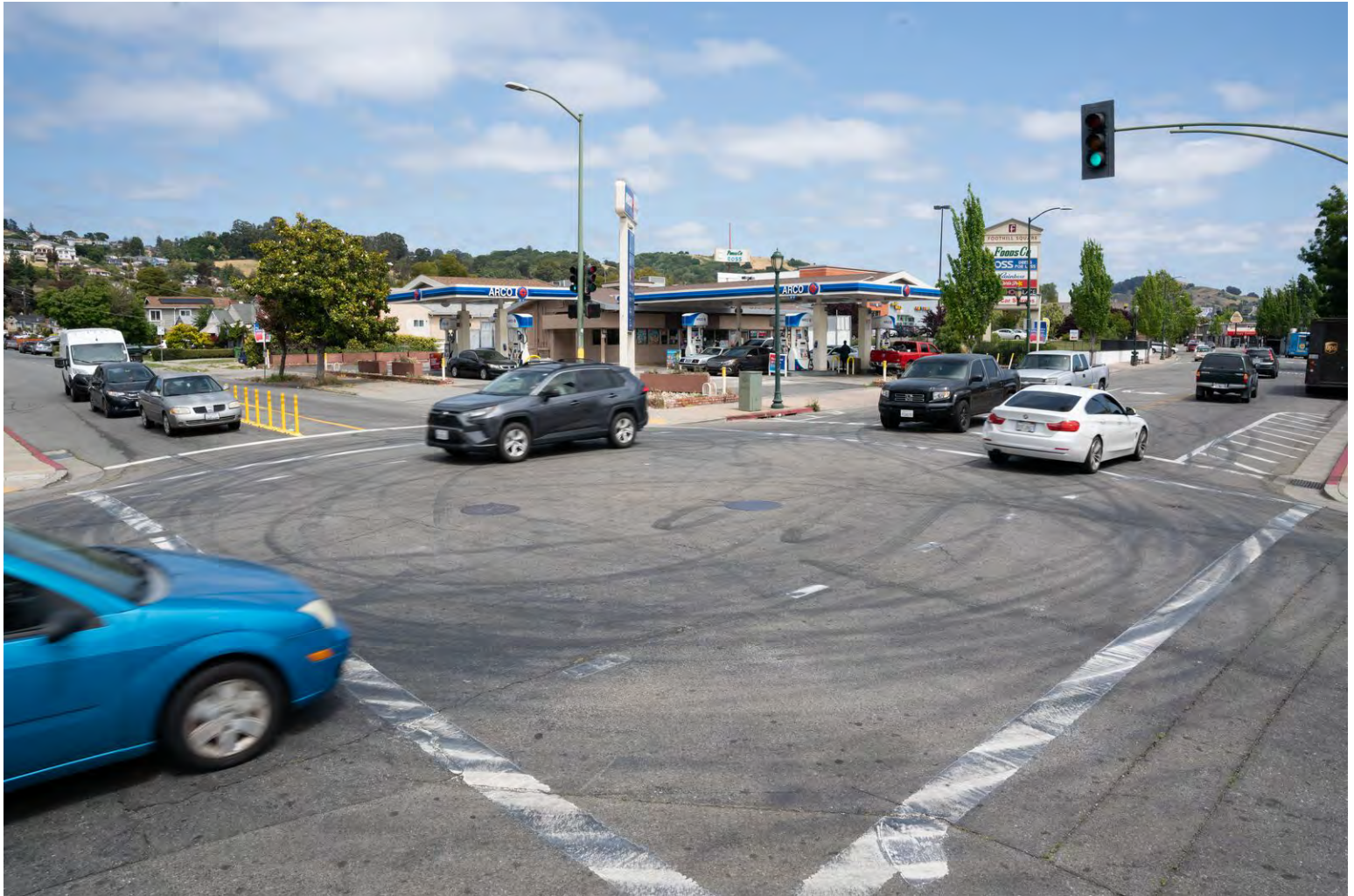
The intersection of 106th Avenue and MacArthur Boulevard was ranked second for the number of sideshows that happened there among all city intersections in 2022. Credit: Florence Middleton
